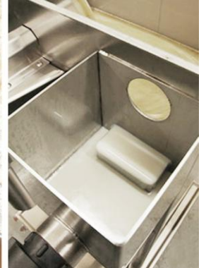
Clean coolant returned to sump
